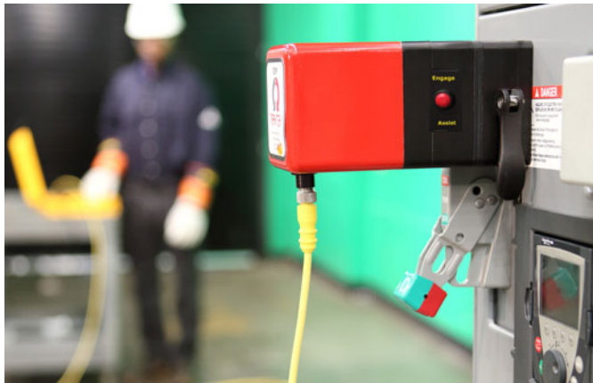
Motor Control Center Bucket Racking Device
